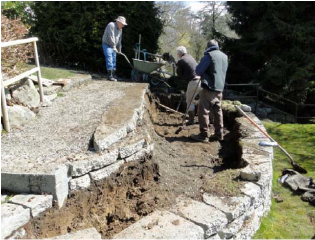
Excavating the bed. Photograph by David Sellars.
