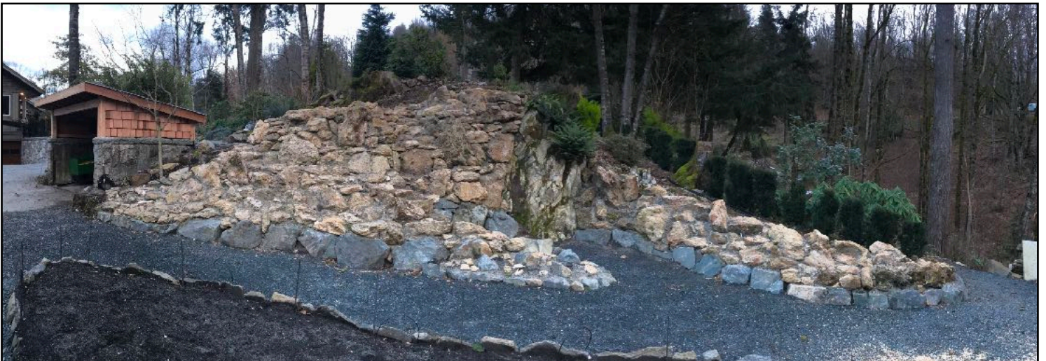
Below: Current view of project.
