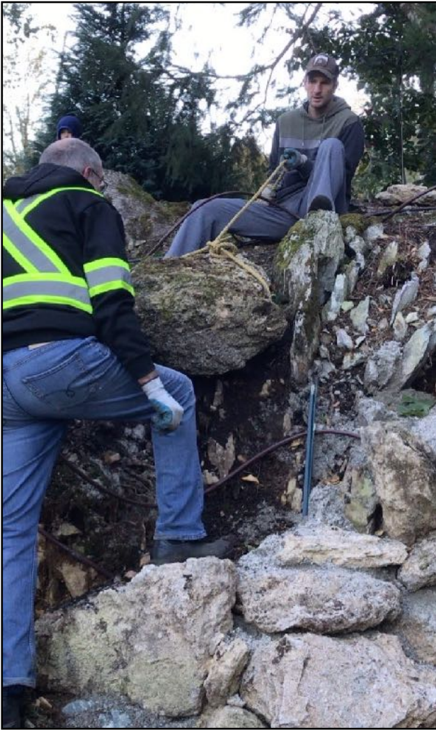
Above left: Placing large boulders around irrigation lines.
