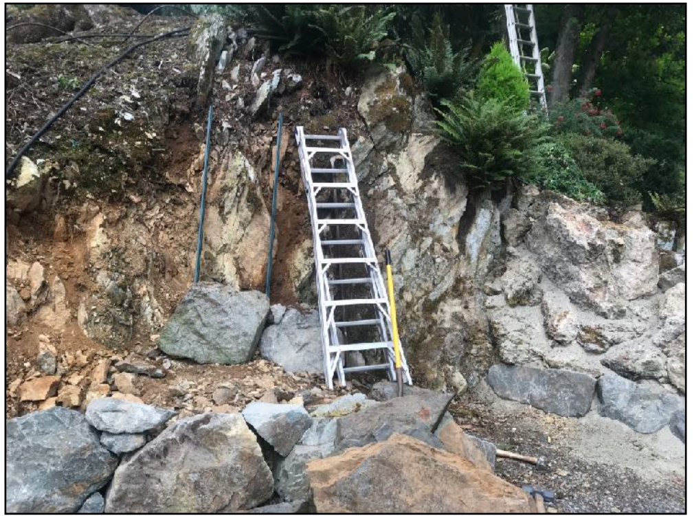
Placement of boulder base.
